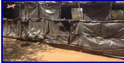
temporary pole frame made of tree branches and fastened sheets of sheet metal to it, forming a makeshift roof as shelter from the rain
